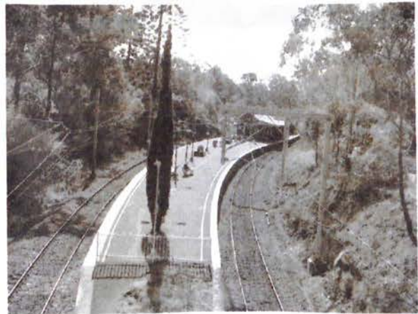
(Beecroft Station as it is now - north of the Copeland Road crossing)
